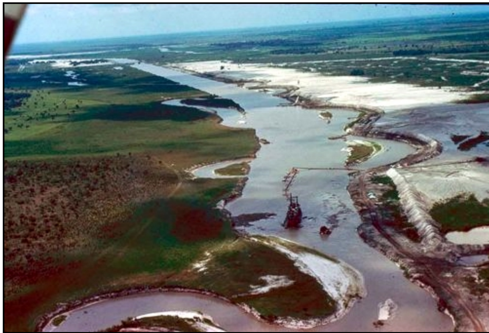
Construction of C-38. (Source: U.S. Army Corps of Engineers, Jacksonville District.)
