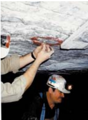
Attaching a plumb bob string to a spad.
