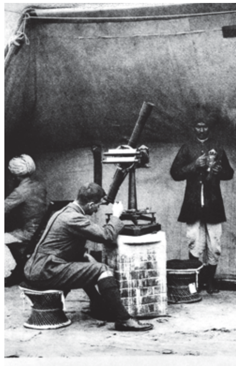
Figure 3-14: Astronomical observations were used in early geodetic surveys to measure datum locations (courtesy NMSI)
