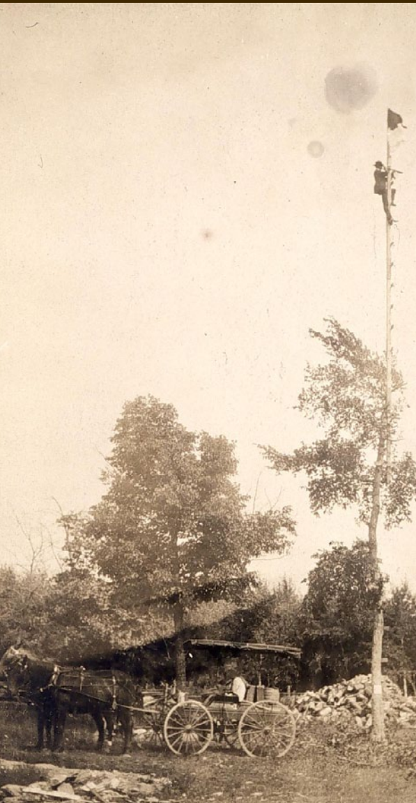
A 1903 photograph of Jasper Bilby atop a "guyed pole" performing reconnaissance in order to properly place a wooden tower. Hmmm, there's got to be a better way.
