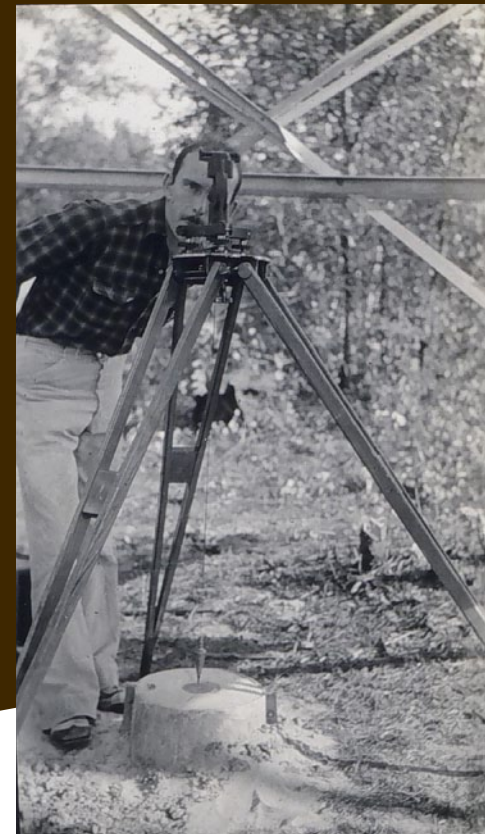
How did they center a 95-foot tripod over a point? Carefully plumbed, a vertical sighting device was used to center the transit mount high overhead.
