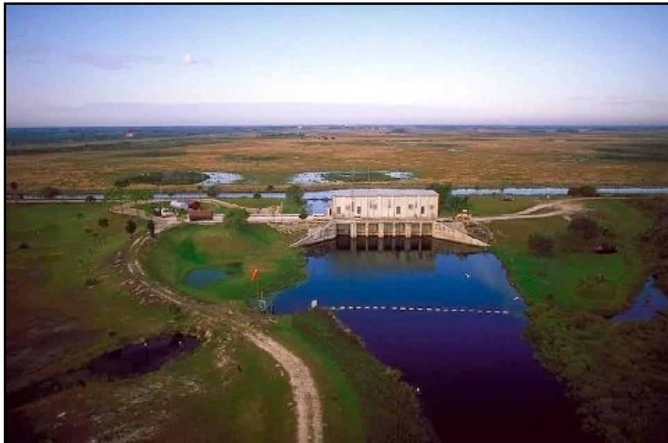
The S-140 pumping station. (Source: South Florida Water Management District.)
