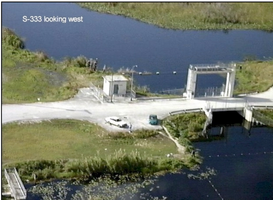
S-333 looking west. (Source: U.S. Army Corps of Engineers, Jacksonville District.)
