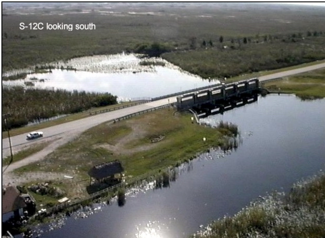
S-12C looking south into Everglades National Park. (Source: U.S. Army Corps of Engineers, Jacksonville District.)
