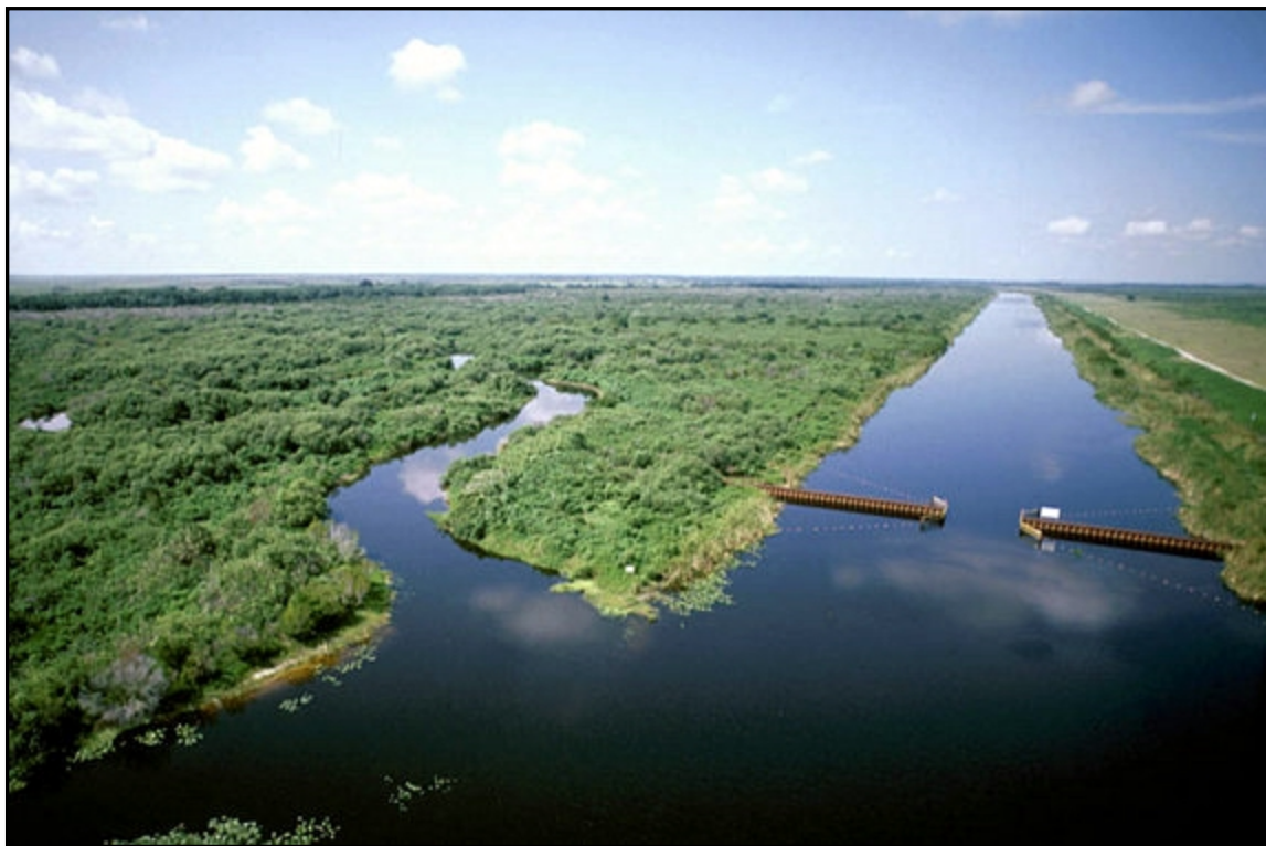
Weirs placed in the Kissimmee as part of the Demonstration Project. (Source: South Florida Water Management District.)
