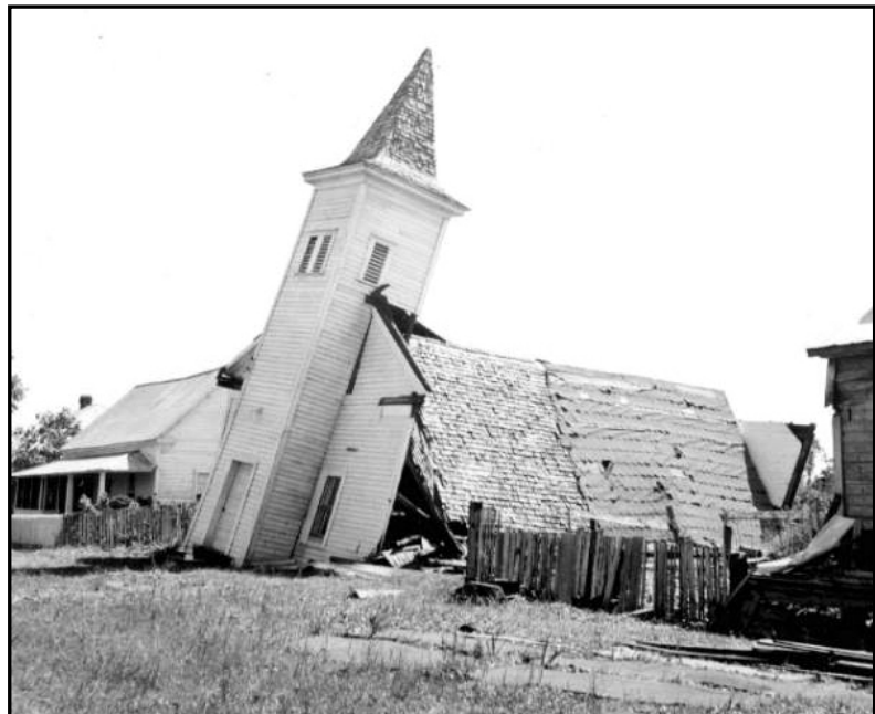
Damage caused by the 1947 hurricane. (Source: The Florida Memory Project, State Library and Archives of Florida.)
