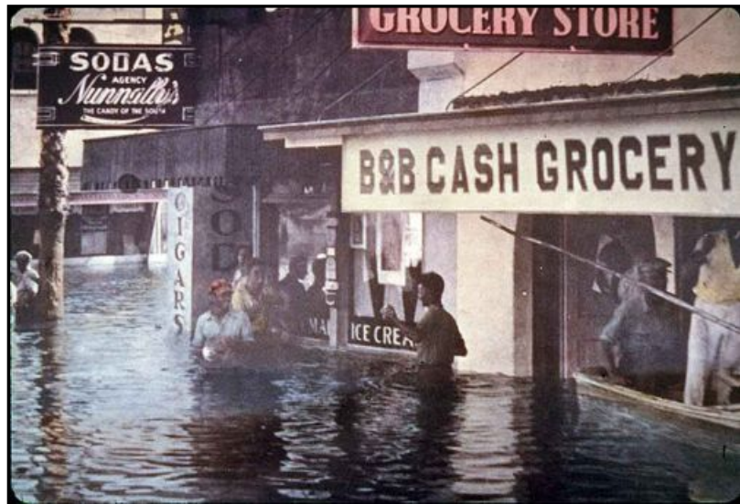
Flooding from the Kissimmee River in the town of Kissimmee. (Source: South Florida Water Management District.)
