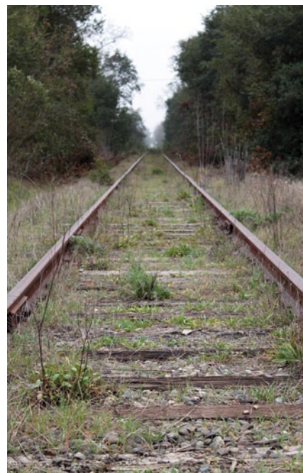
The existing Northwestern Pacific railway corridor will soon be a modern, passenger rail system.
