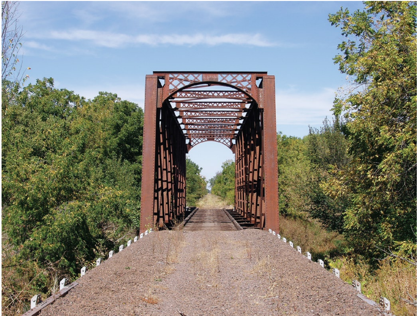
Bridges such as this one are often all that is left to define the location of the centerline where the track once existed. (All photos by Jerry Penry)
